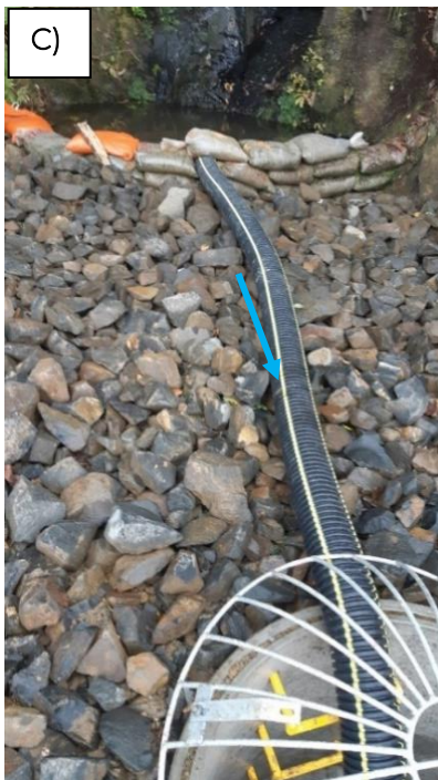
Figure A3. Site G2 (CH12980): A) waterfall and stream upstream of the road, B/C) current installed inlet with large rip rap with subsurface flow to scruffy dome, D) current outlet showing perch.
