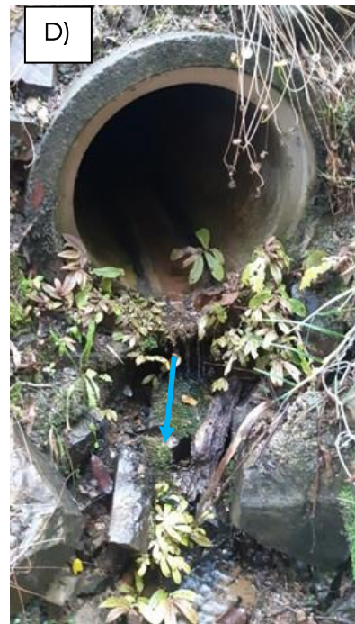
Figure A3. Site G2 (CH12980): A) waterfall and stream upstream of the road, B/C) current installed inlet with large rip rap with subsurface flow to scruffy dome, D) current outlet showing perch.
