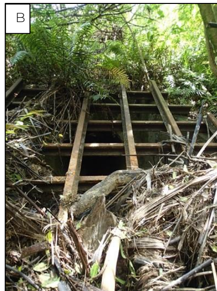
Plate 3-9: A) Stream at Site I, upstream of SH1 in December 2023, B) Culvert inlet with large debris screen.
