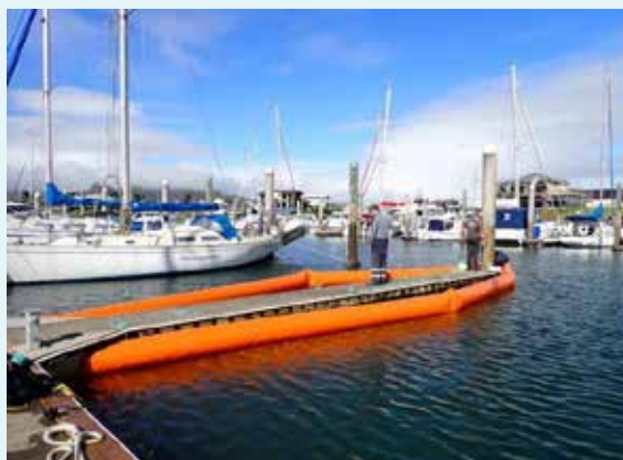
A berth at Marsden Cove Marina fully encapsulated with a weighted turbidity curtain
