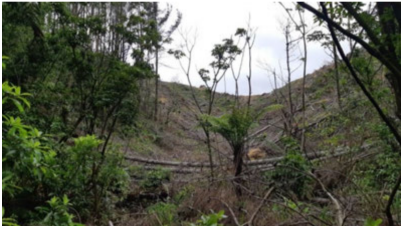
Photo 15: Site B1 Upstream: Wetland and stream upstream of the road prior to construction in December 2024. This shows the recently semi-felled exotic forest. This wetland complex and stream habitat was completely reclaimed by fill area B.
