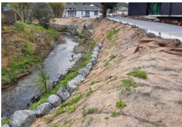
Right of photo: Coconut matting used for riverbank protection.
