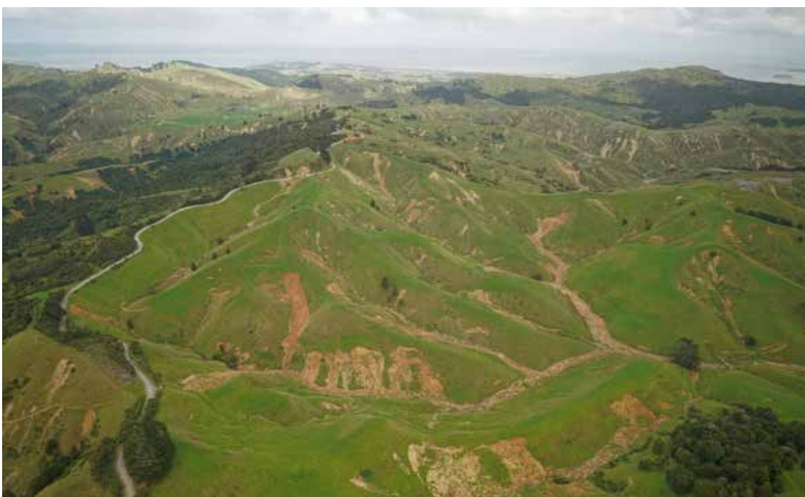
Extensive slip and gully erosion in the Kaipara Harbour catchment following Cyclone Gabrielle in 2023. Source KMR.
