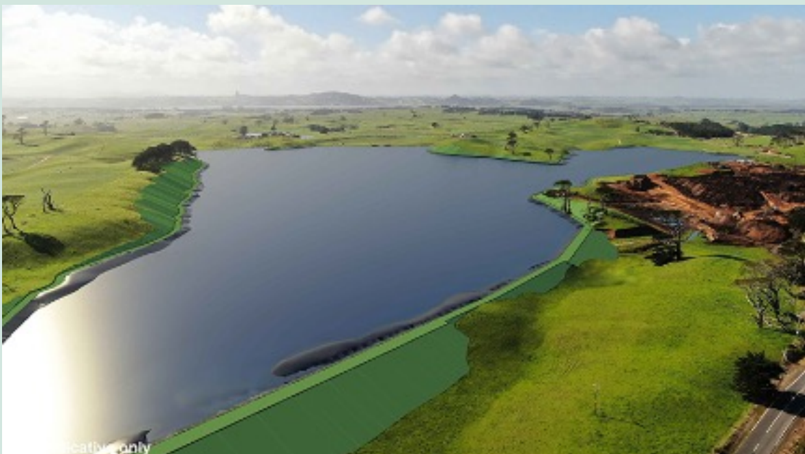
Artist's impression of a completed Te Waihekeora reservoir on the Pōuto Peninsula. Source: taitokerauwater.com/kaipara
