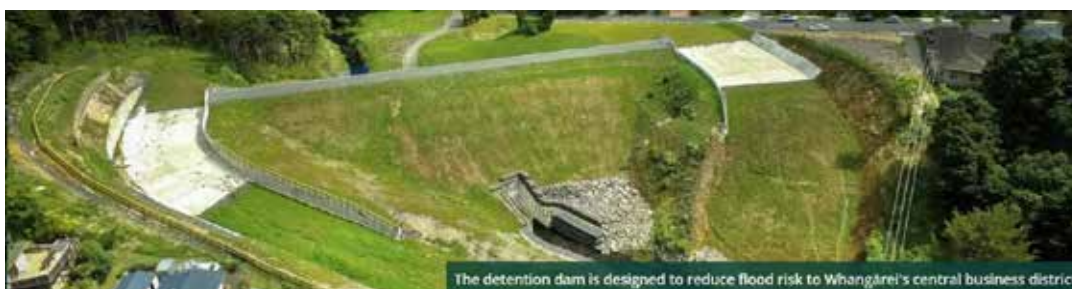
The detention dam is designed to reduce flood risk to Whangārei's central business district.
