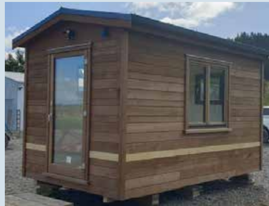
Cabin built with Kawa poplar as part of Northland Regional Council's research into opportunities for the Kawa poplar cultivar. Source: NRC.
