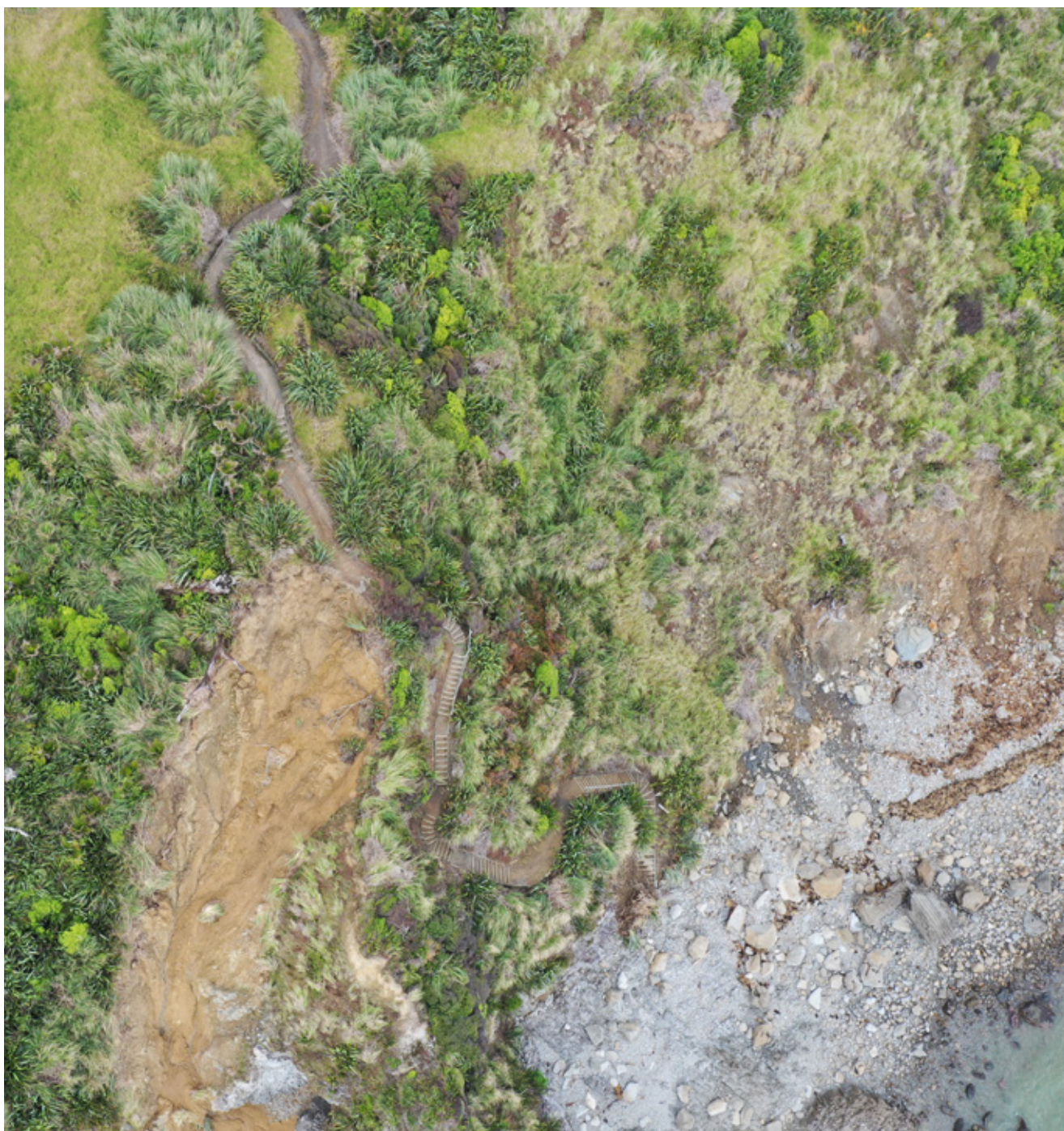
Eroded section of the Mangawhai Walkway
