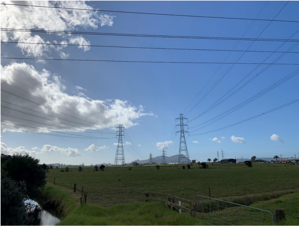
Figure 4: Showing offset site (Site 3) facing north from Mccathie Road (26 July 2024)
