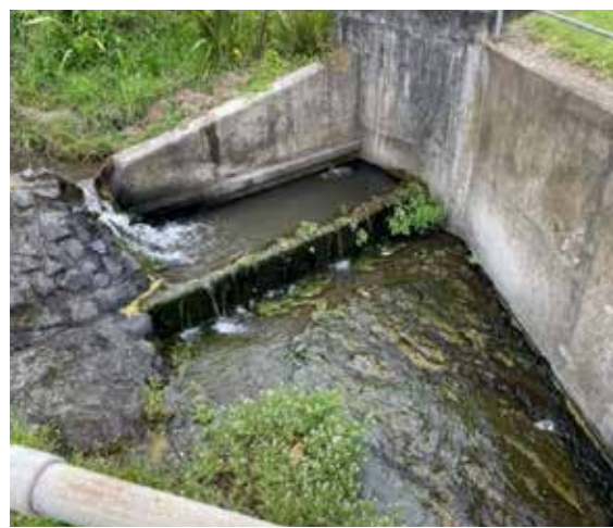
A fish barrier structure at McLeod Bay. Īnanga were found in the concrete pool (centre of image), but not upstream of the weir (centre left of image).
