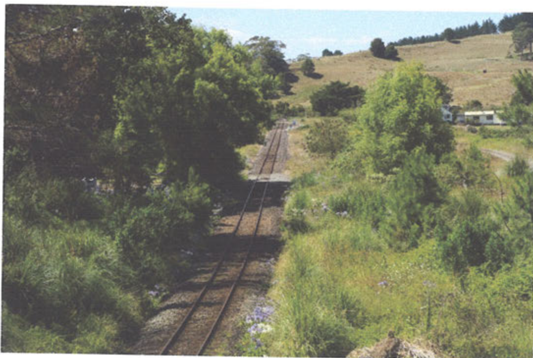
Photo is looking north east from Highway Over Bridge to where Junction will be built, 3km south of Wood Chipping Plant that would connect to Marsden Point, Forms Part of a Network 1,800 South to Bluff via Cook Strait Rail Ferry, LONG TERM Advantages Out Weigh Current short term Cheap Truck Fuel
