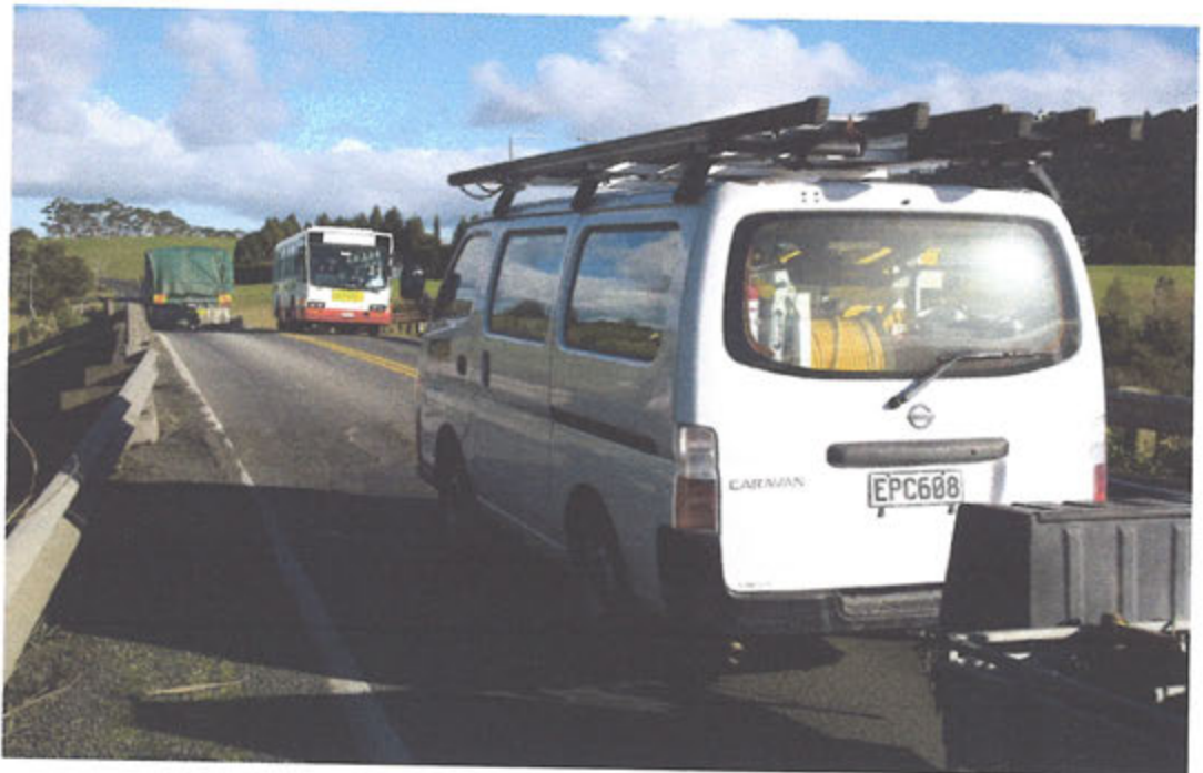
Photo is Looking South between Apotu Rd intersection and Bridge, NOTE Narrowness of Bridge, NO Cycle Margin, Width of "Over width" truck and Closeness to the School Bus, DANGEROUS "NETWORK FIT"
